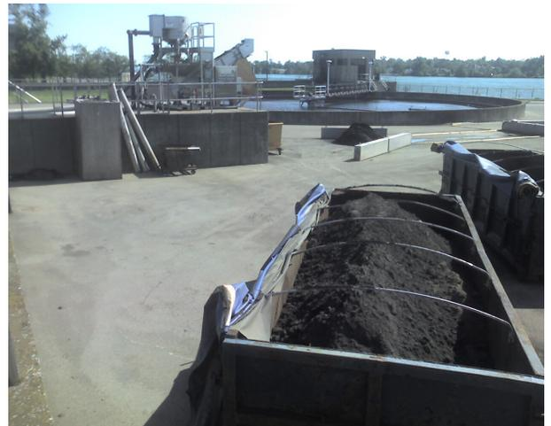
*Grit Removed from Sludge by SlurryCup / Grit Snail*
