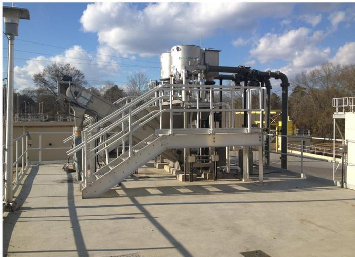
*SlurryCup™ / Grit Snail® Sludge Degritting Solution*
