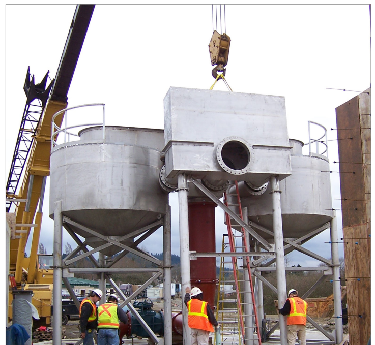
Chehalis Grit King® System During Installation
