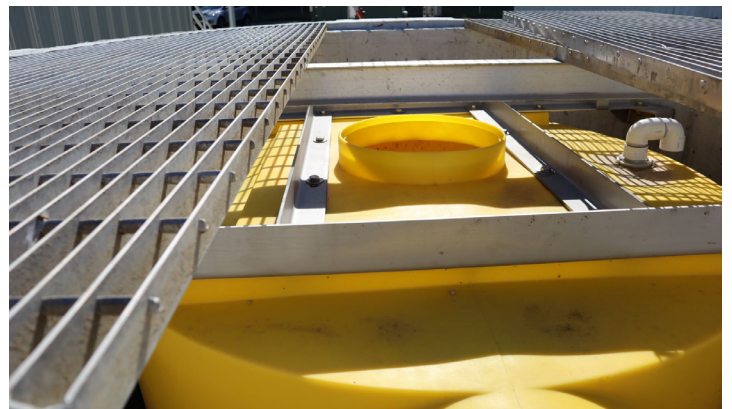
Shiloh's installed Grit King® Compact
