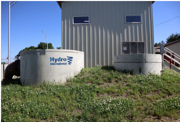
Shiloh's installed Grit King® Compact (left) and grit pump chamber (right)
