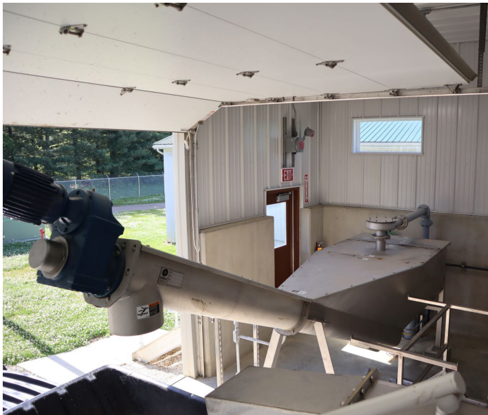
Underflow from the Grit King® is sent to a screw classifier for dewatering.
