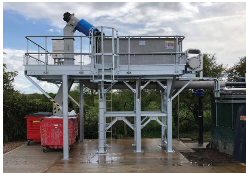
The MNSS Combined Screen combines screening, washing, transport, compaction, and dewatering in a single cost-effective standalone solution.
