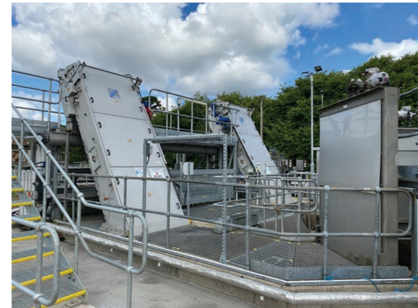
The robust FSM Filterband Screen delivers fine screening of sewage and sludge with no requirement for coarse screening upstream.
