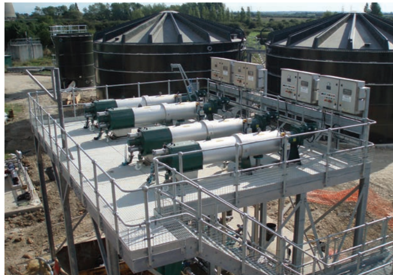
The small-footprint, low maintenance Hydro-Sludge™ Screen is ideal for small works with no inlet screens or for screening of tankered sewage.
