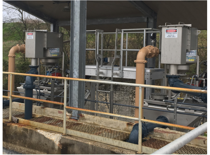
TeaCup® / Grit Snail® Systems with Standard Discharge Box Design
