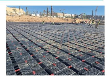
At the site, the team prepared the excavation with a geotextile and sand/gravel levelling layers. The lightweight crates were then placed by crane and "snapped" together – a process Hydro International notes is "quick to install" for such modular systems.
