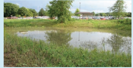
Fig.3 FAA regulations prevented installing a larger pond because it would have attracted waterfowl; a hazard to aircraft. The filter allowed the airport to continue relying on its small detention pond.
