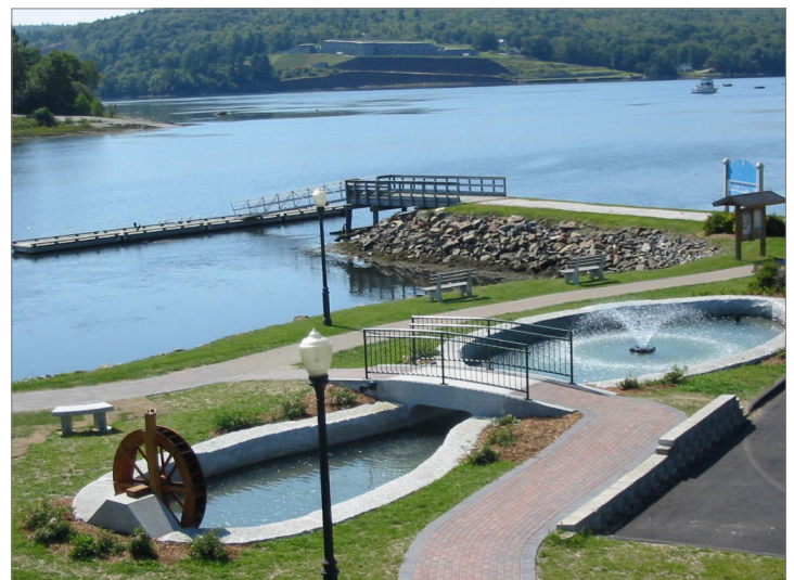
Exterior View of CSO Facility and Fort Knox (Across the River)
