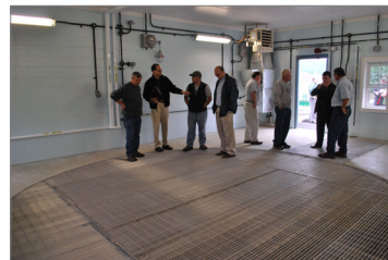
Interior Storm King® Facility
