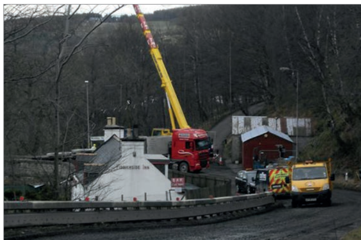
Chamber offloading on site.
