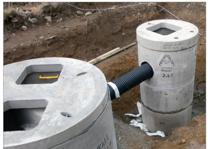
Hydro-Brake® Flow Controls and Downstream Defender® during installation on site.
