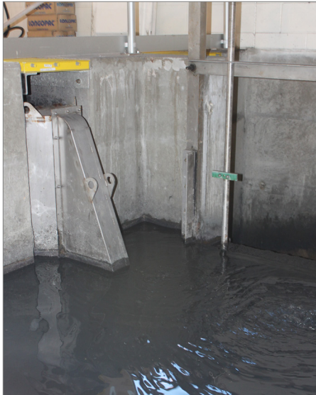
Operating HeadCell® Submerged in Tank (inlet duct is visible on the left)
