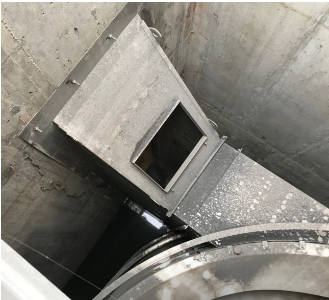
HeadCell® inlet duct mounted to inner tank wall
