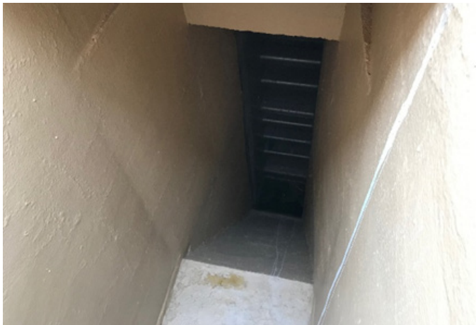
Formed transition from inlet channel
