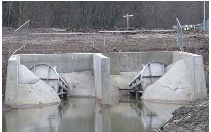
The finished installation.
