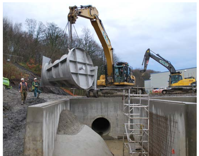
One of the two Hydro-Brake® Flow Controls being craned into position.
