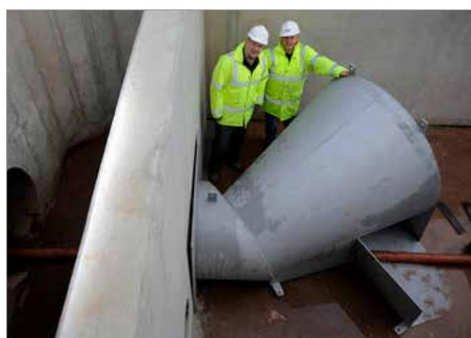
"Compared to alternative flood control devices such as orifice plates or penstocks, the vortex flow controls have a larger opening, so more water is able to flow through the culvert unimpeded, meaning less flood storage is needed. At the same time, there is less risk of blockage. This, together with the fact that the flow controls have no moving parts or power requirements, means they require minimal maintenance."
