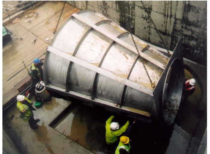
The Hydro-Brake® Flood flow control during construction
