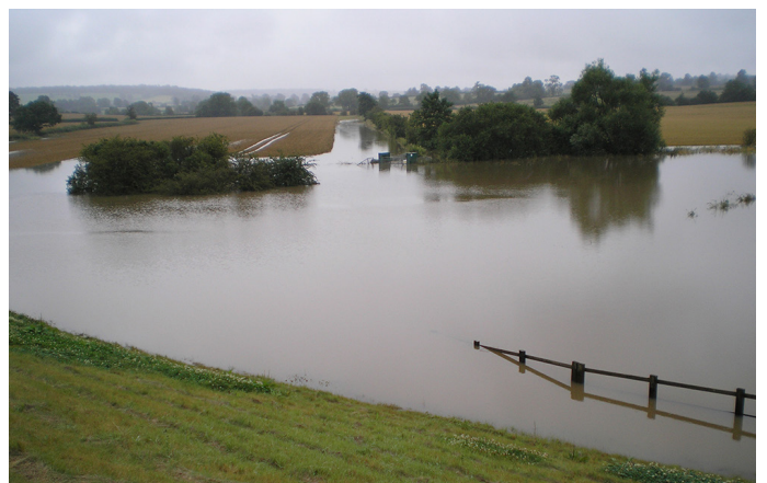
The flood storage area in use following storm conditions
