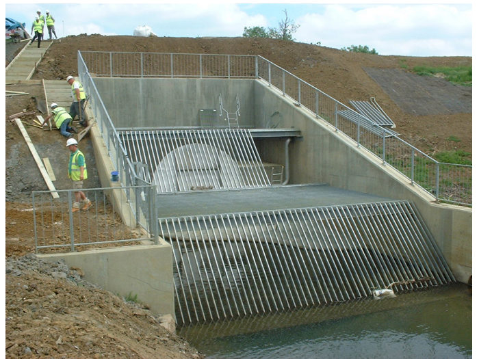
Construction of the trash screen
