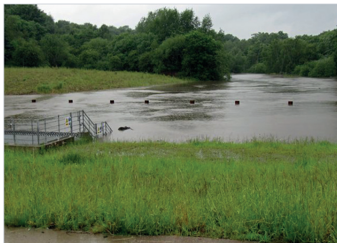
The flood storage area behind the Wigan dam.
