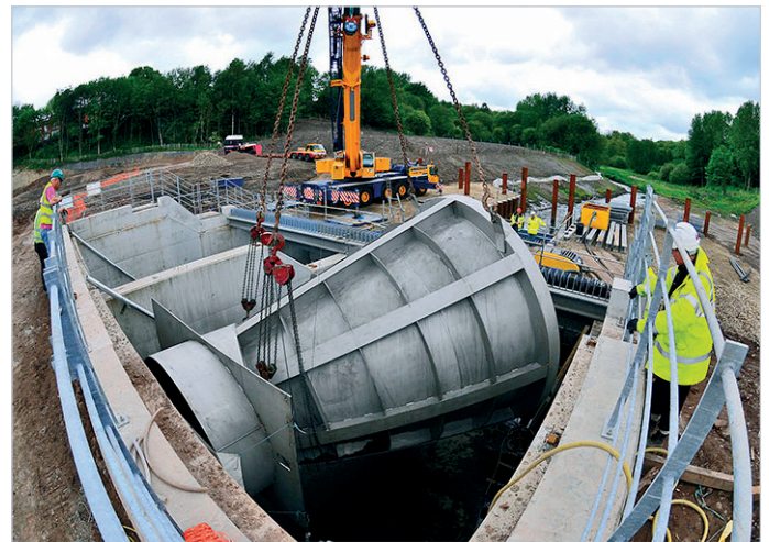
Installation of one of the Hydro-Brake® Flood vortex flow controls.
