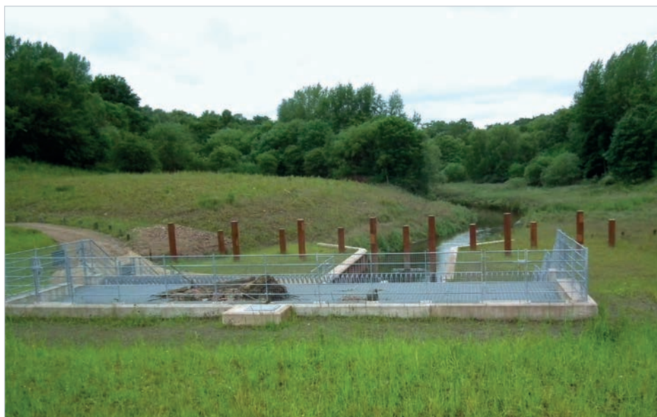
Landscaped area after installation
