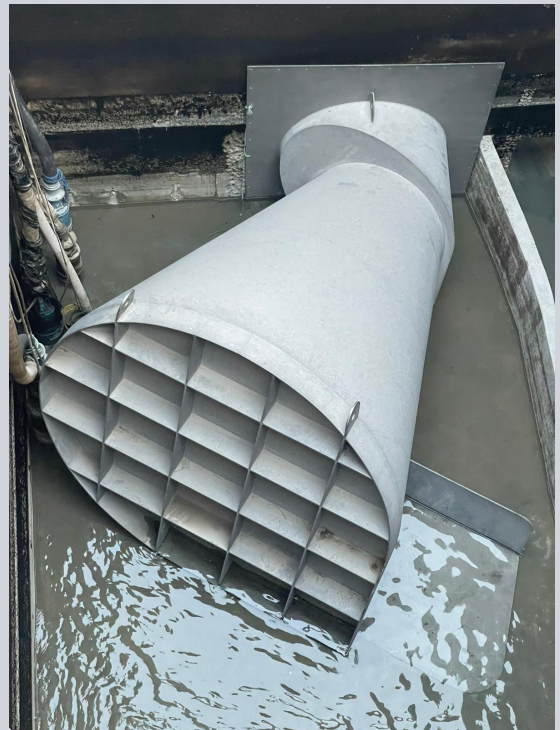
*Supplied Hydro-Brake® Flood during installation
