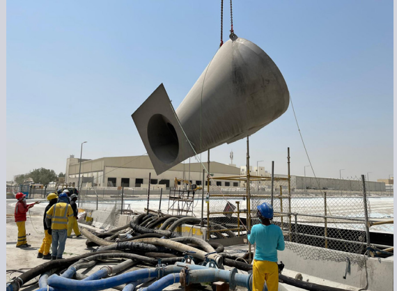
*Supplied Hydro-Brake® Flood during installation
