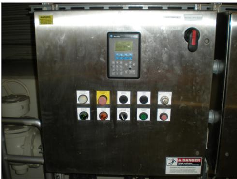
Improved PLC control panel with HMI
