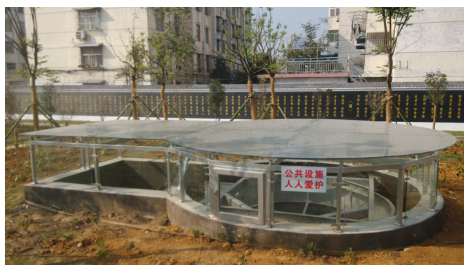
Unusually, the Storm King® system was installed above ground in a public park, to raise awareness of the water quality improvement project
